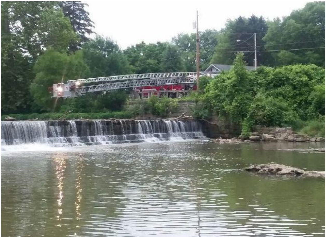
A Findlay Fire Department truck extends its ladder out over the Blanchard River from the south side, Friday at Riverside Park. The exercise was done to test how far the department's ladders can reach across the river during a water rescue, recalling efforts to rescue two teenagers from the swollen river in 1978 that saw two firefighters lose their lives. (LOU WILIN / The Courier)
