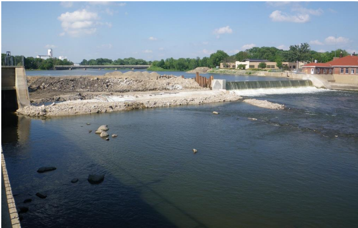
Photo above during reconstruction on 7/30/2011
