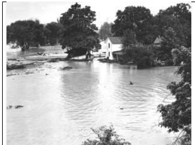
Smashed buildings show the damage caused by flood water from the Little Apple Creek that swamped the area around Bauer Rd. in Wooster, OH. Photo courtesy of Vicki Slater.
