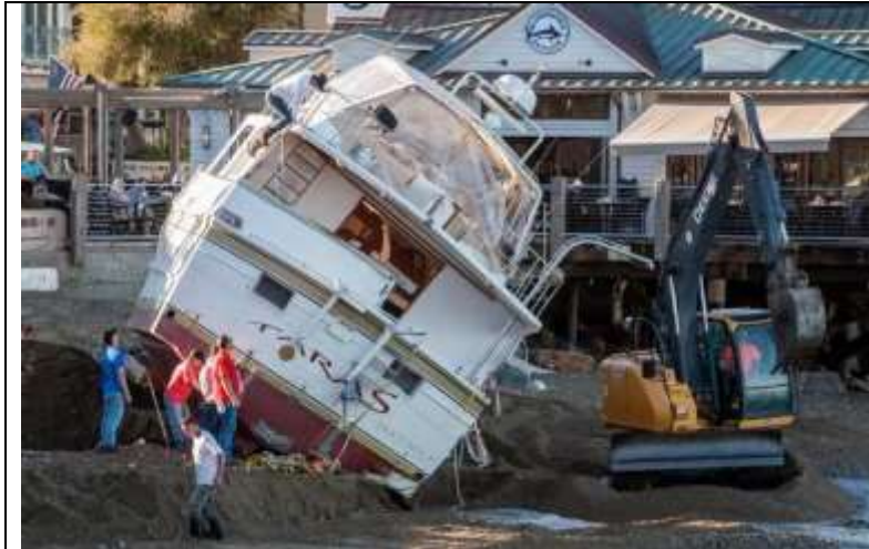
Workers and earth-moving equipment dig a moat around a boat stranded on the beach in Avalon on Catalina Island on Tuesday, in order to float it off the beach at high tide.
